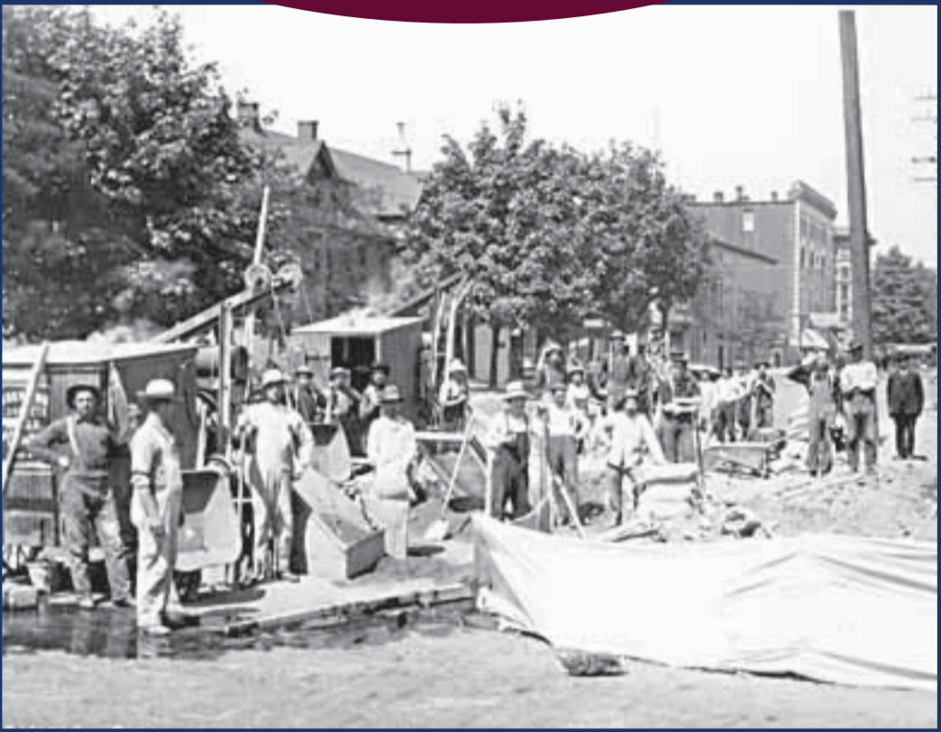
G.W. Ledingham, Contractor Laying Cement Sidewalks [500 block Georgia St] -- [190-?]
